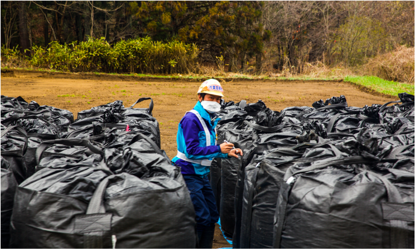
Figure 1. Worker at radioactivity decontamination site near Fukushima labeling bags filled with topsoil removed from contaminated areas. Image credit: Andrew R. Marks.
